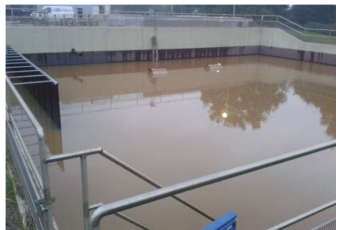
Before OLOID installation
