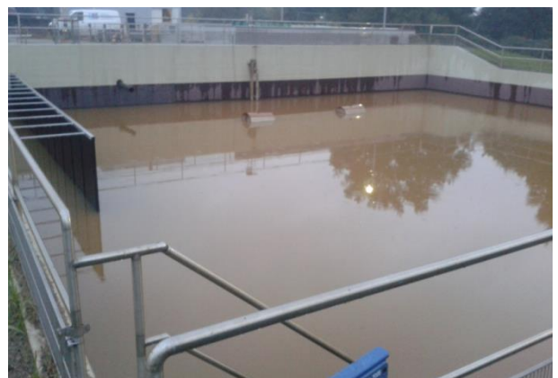
Before OLOID installation
